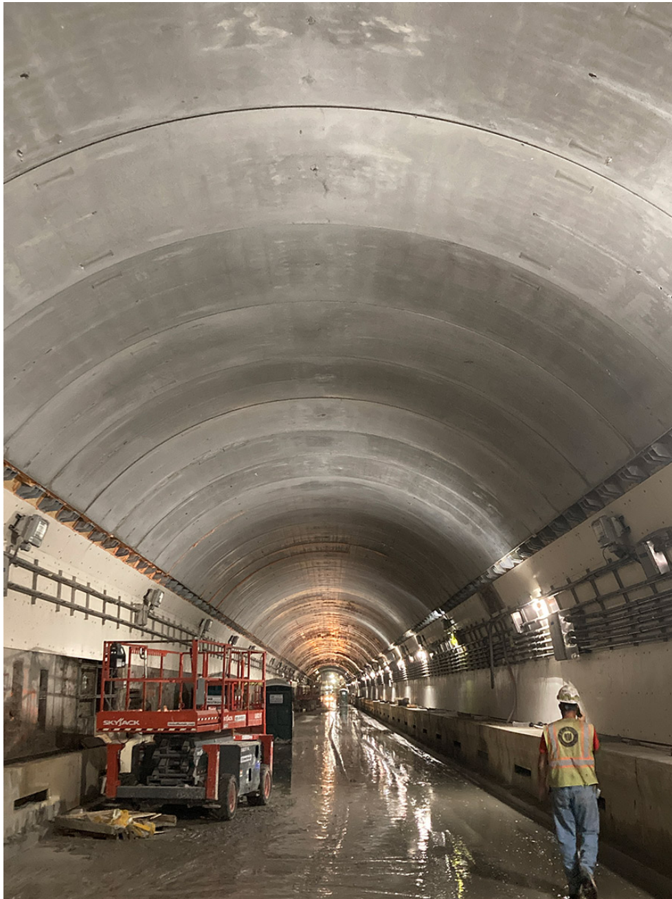
New precast concrete arches, freshly installed
