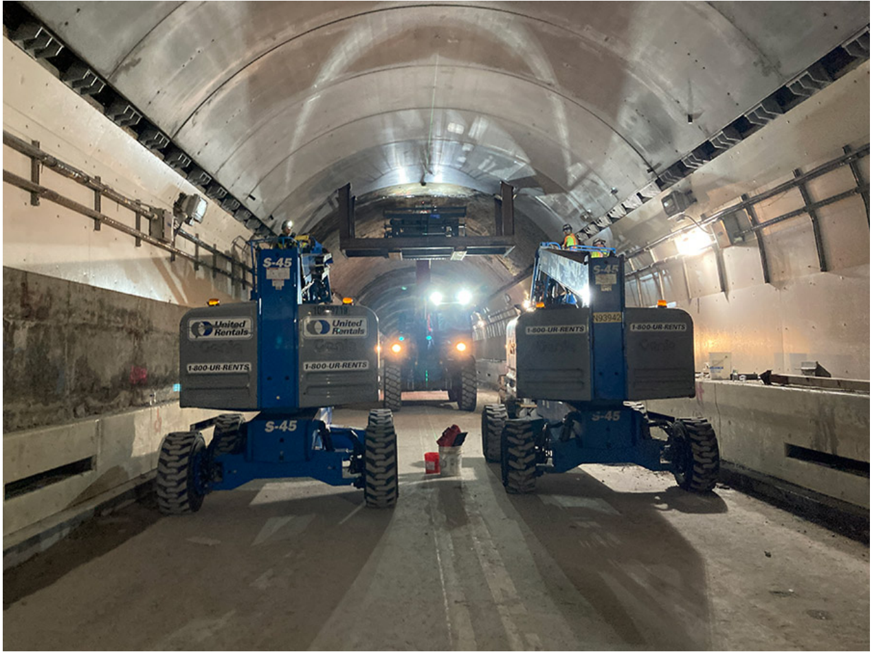
Precast arch panel being put into place.
