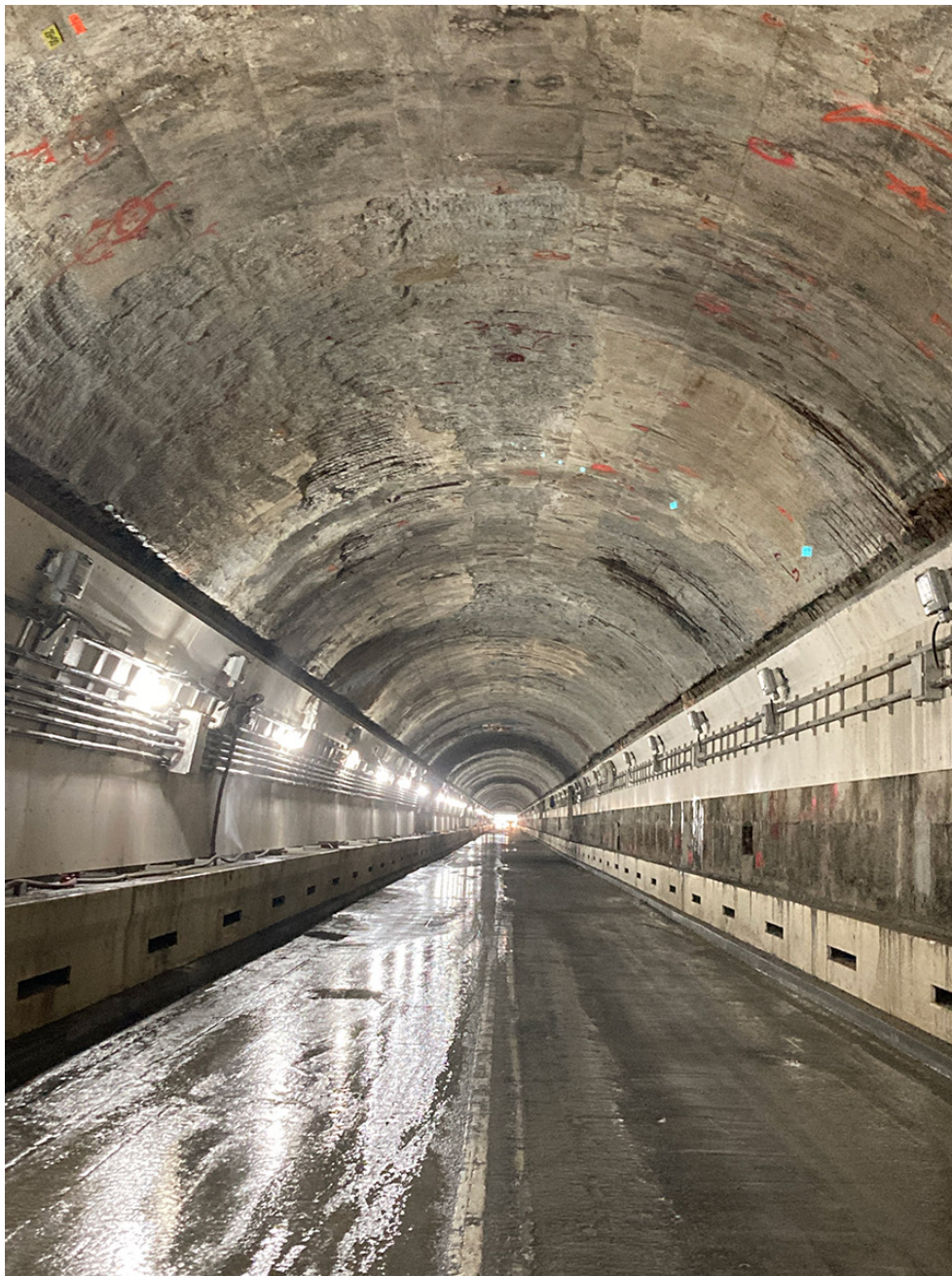
Existing tunnel ceiling, ready for precast installation
