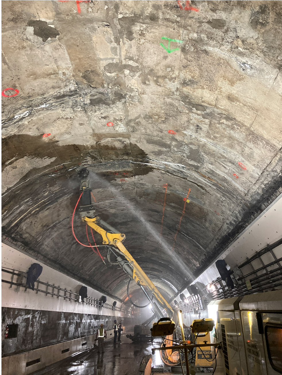
Preparing existing concrete ceiling for precast arch installation
