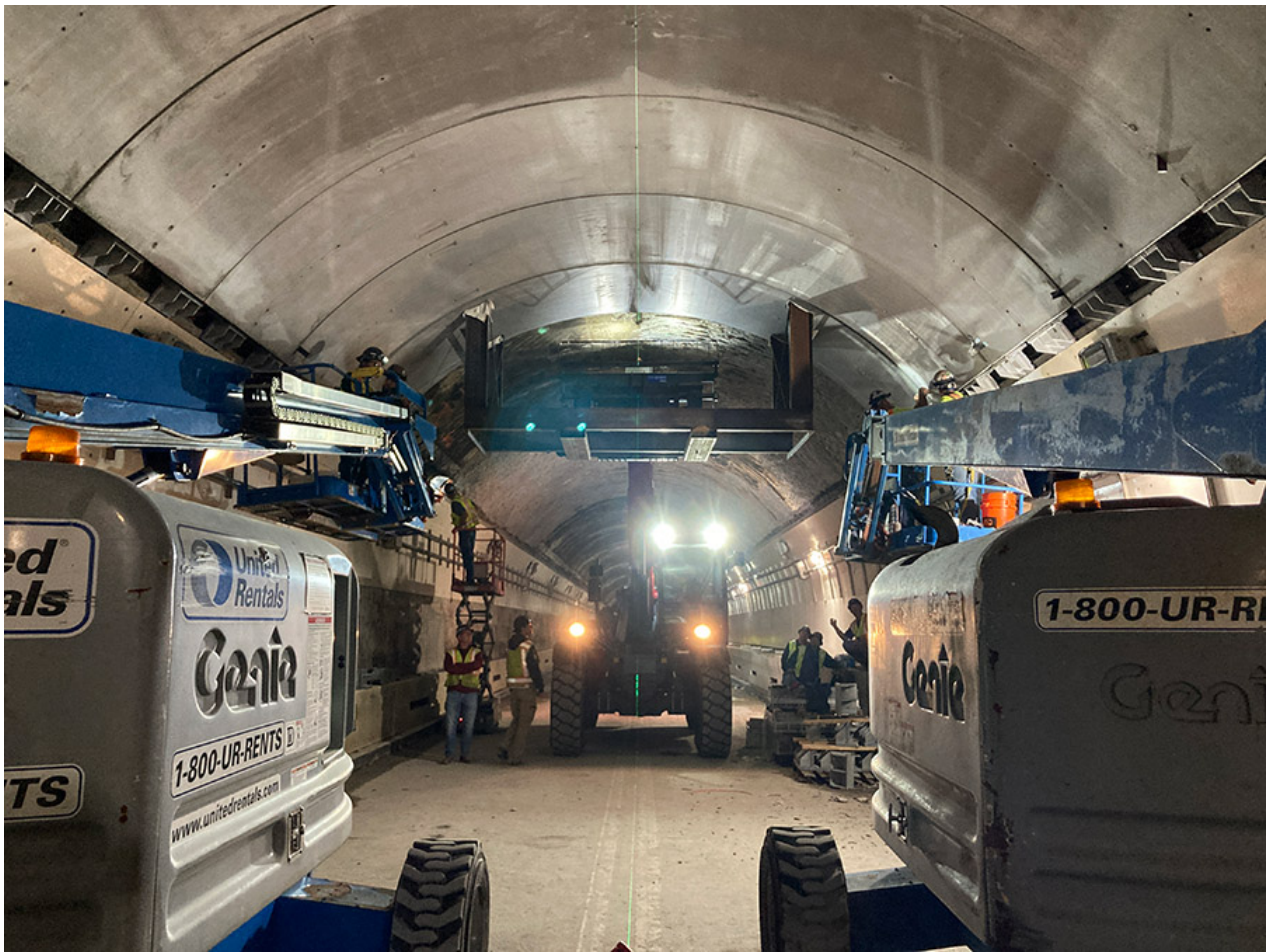
One of 783 precast concrete arches being put into place.
